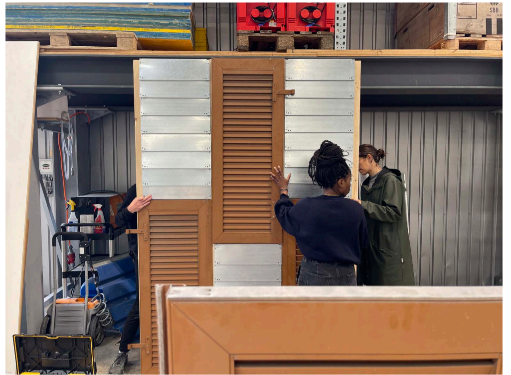
construction of facade modules
