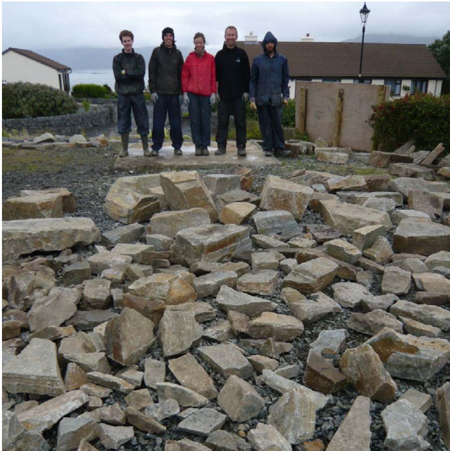
Fig. 4 Catagorizing the stones, Drystone Workshop, Ireland, 2009.
