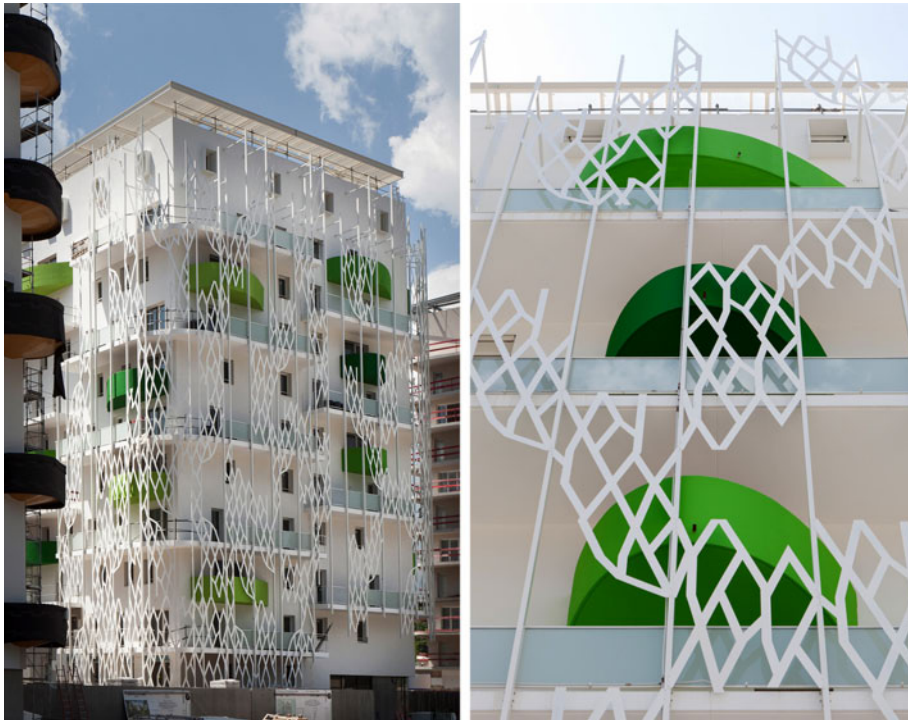
Fig. 5 Bio-inspired building skin (in collaboration with GTB Architects).
