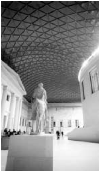
Fig. 27. British Museum Great Court Roof, Foster and Partners, Buro Happold, Waagner-Biro
