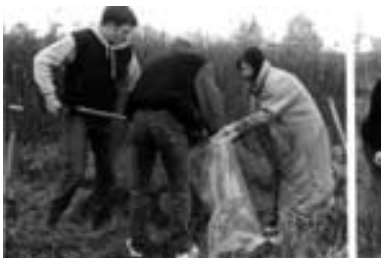
Loading earth to marked sacks
